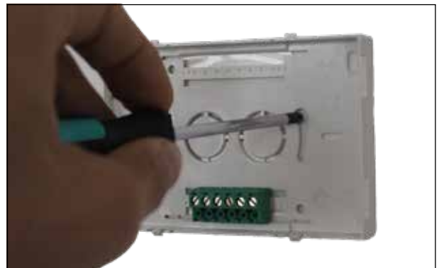
Screwing the installation board of the gateway
