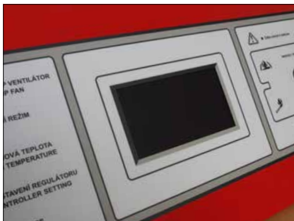
Controller installed in the boiler instrument hood
