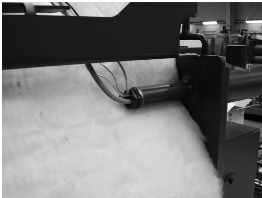
WF boiler temperature sensor in a pocket, added to the other sensors of thermostats of the original electro-mechanical control of the boiler
