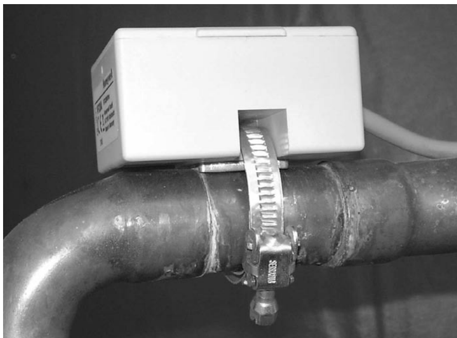
Contact sensor after the mixing valve to the heating circuit
