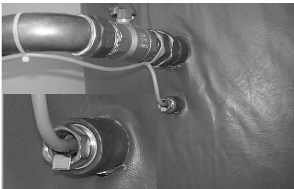
PF temperature sensor of the top part of the tank (VE), or DHW sensor in a combined DHW heater inserted in a pocket . !!! The PF sensor (VE) must always be at least 10 cm under the connection of the pipeline to the tank; we do not recommend you to attach it to the pipeline to ensure optimum function of the controller!!!
