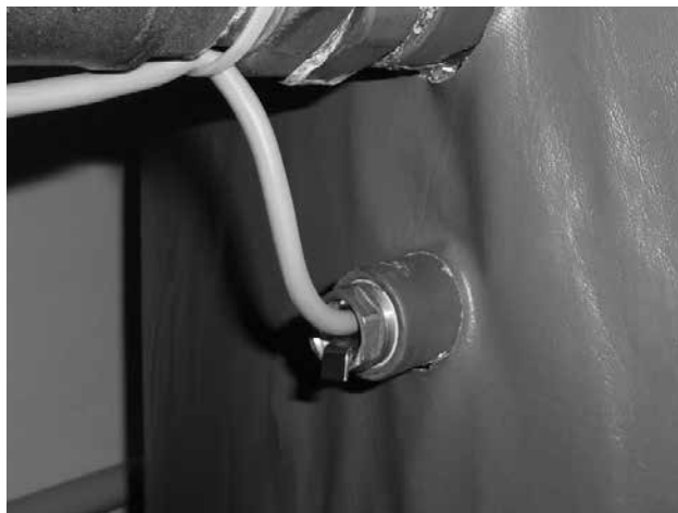
Fig. 14 – View of the water temperature sensor in the pocket of the accumulation tank (TV and TS)
