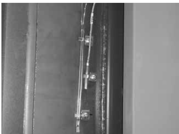
Fig. 15 – a view of the flue gas temperature sensor TSV at the side of the flue gas duct of a DC40SPT, DC40GSP boiler
