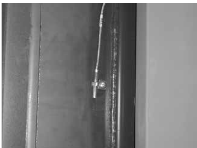
Fig. 15 – a view of the flue gas temperature sensor TSV at the side of the flue gas duct of a DCxxSP(X), CxxSP, ACxxSP boiler
