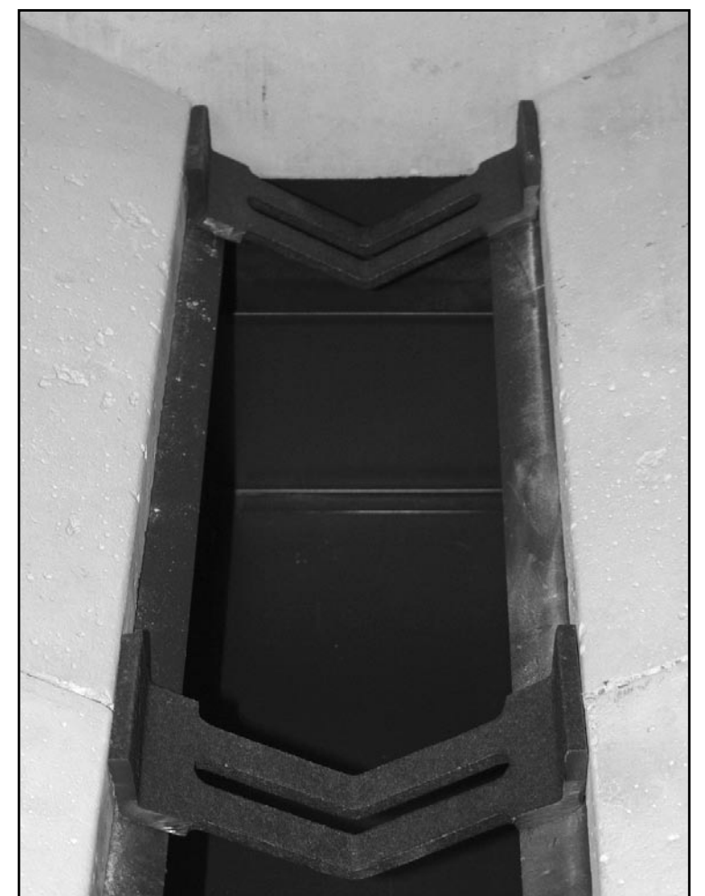
Fitting the holders (spreaders) into the boiler when installing the ATMOS A70 Petro burner.
