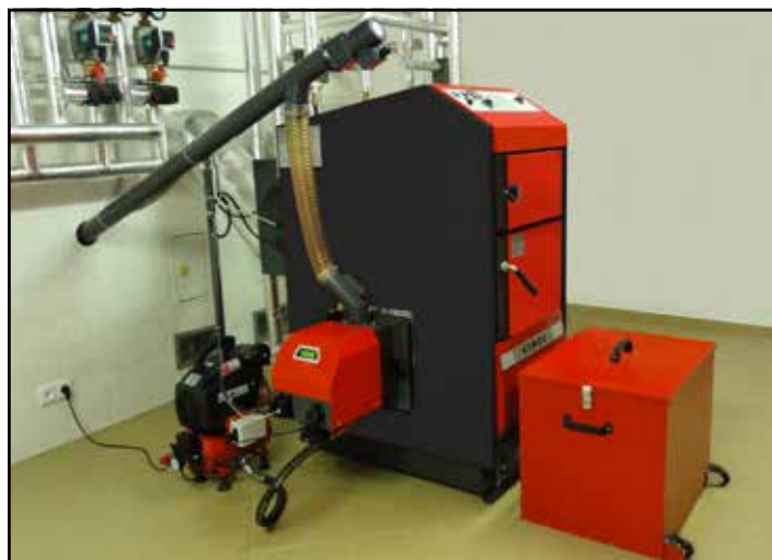
D50P boiler in boiler room
