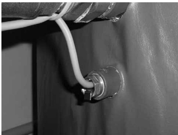
Fig. 14 – View of the water temperature sensor in the pocket of the accumulation tank (TV and TS)
