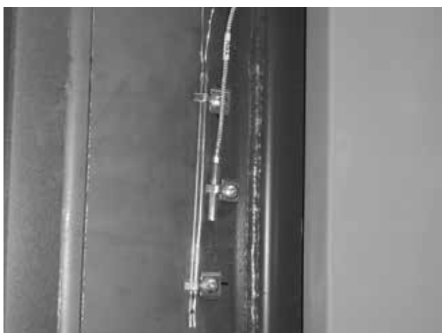
Fig. 15 – a view of the flue gas temperature sensor TSV at the side of the flue gas duct of a DCxxGSP boiler
