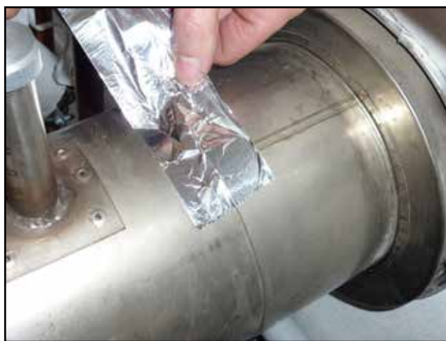
Tightening the flue with an aluminium tape
