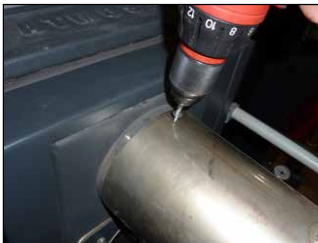
Securing the flue with a screw
