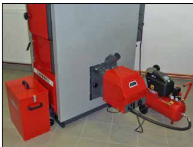
Compressor set up beside boiler
