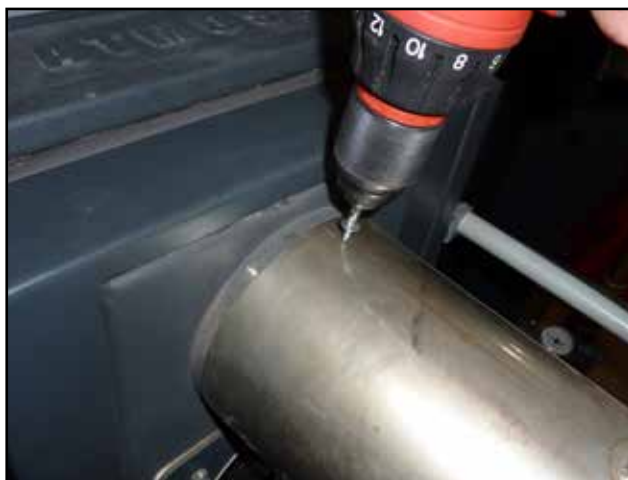
Securing the flue with a screw
