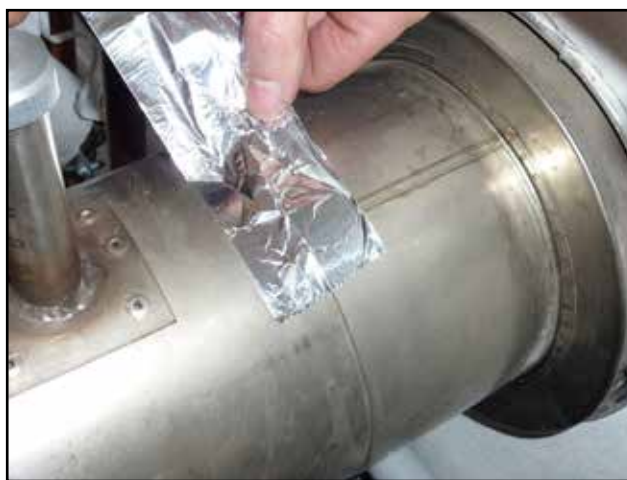
Tightening the flue with an aluminium tape
